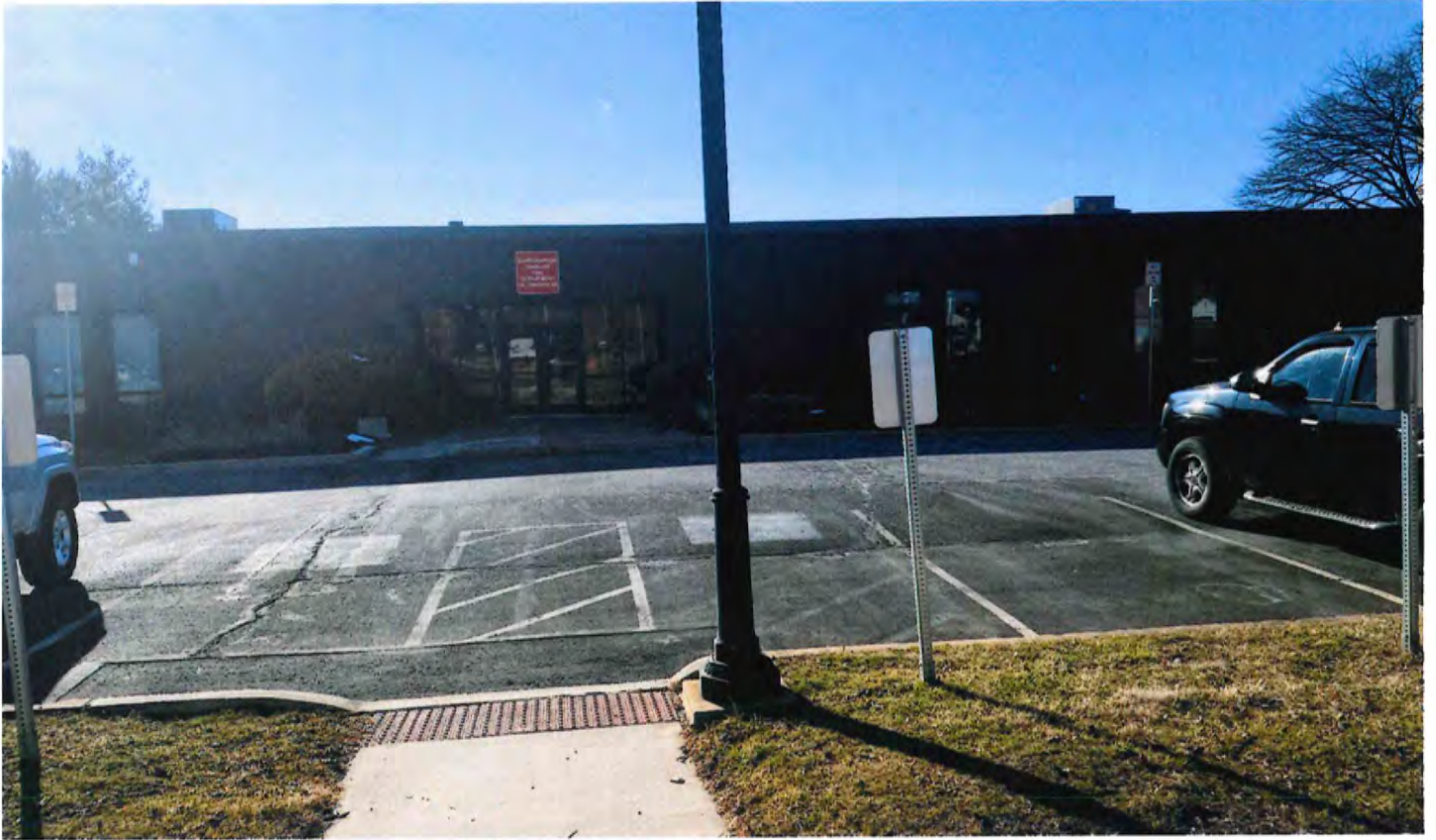
VIEW OF SUBJECT (FRONT-WESTERN ELEVATION)
